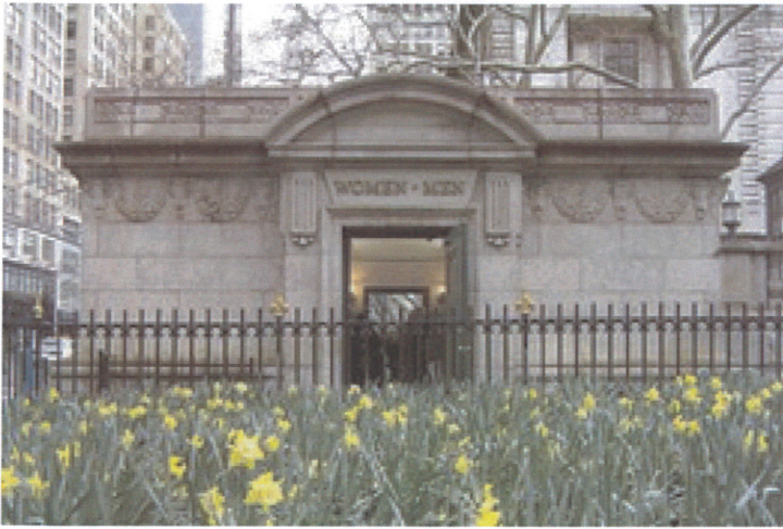
An outside view of the Bryant Park restroom.
